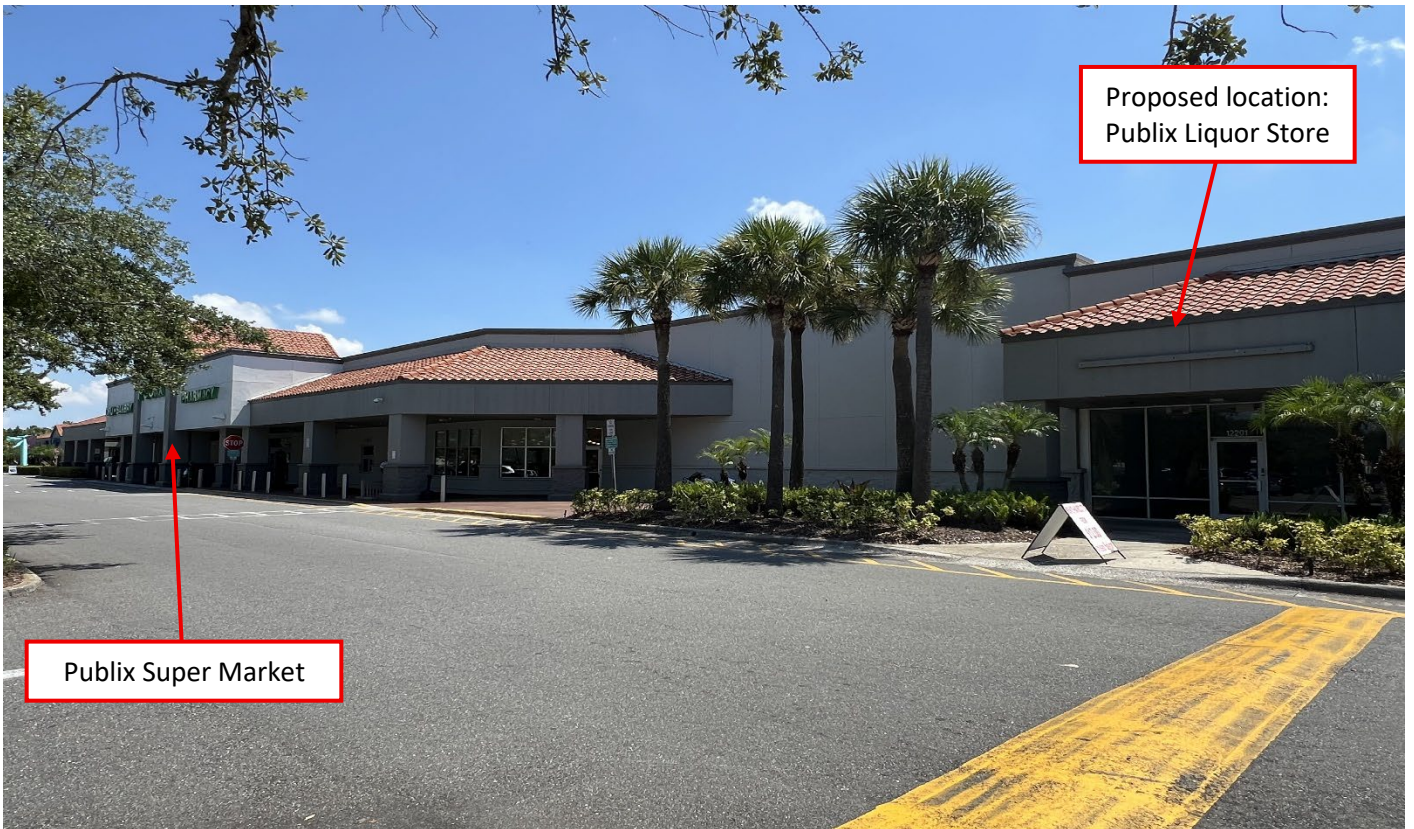
Facing northeast towards subject tenant space
